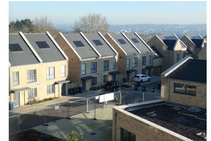
In-built solar panels Image: Well Grove, Christine Johnstone
